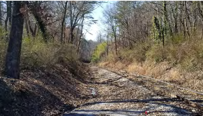
Image shows the Norfolk Southern rail line as travels along Lupton Drive, while ROW is 100-feet wide, the side slopes within the ROW are steep
